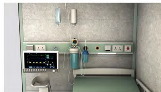
供氧及負壓裝置接入，緊急呼叫終端 Oxygen supply and negative pressure device linked, emergency call
