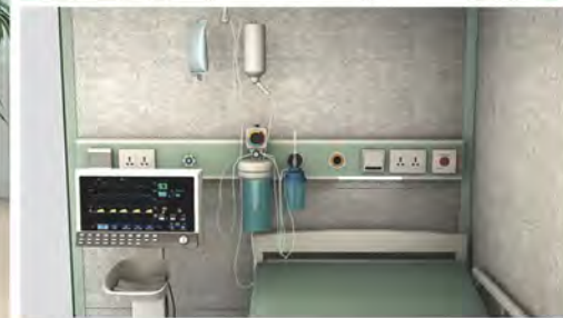
供氧及負壓裝置接入 緊急呼叫終端 Access for Oxygen Supply and negative pressure facilities Emergency call terminal
